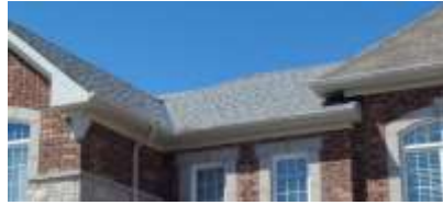
Pic. 2: Roof covering
