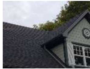
Pic. 3: Roof covering
