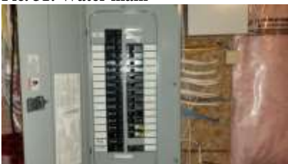
Pic. 34: 100 amp breaker panel
