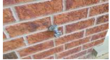
Pic. 6: Hose bib shut off
