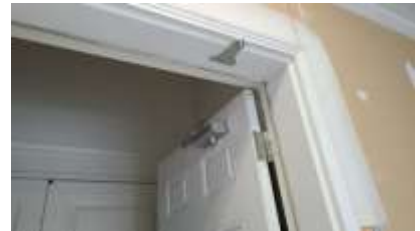
Pic. 9: Auto closer for garage entry door need to be reattached
