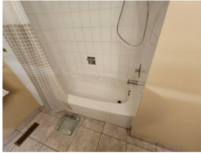
Pic. 17: 2 nd floor bathroom
