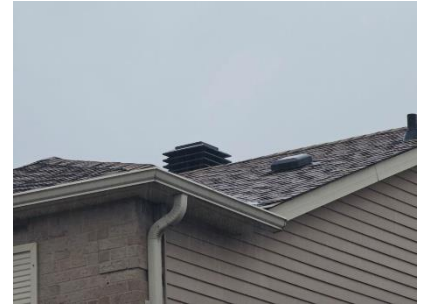
Pic. 3: Updated roof covering
