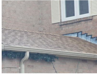
Pic. 2: Updated roof covering
