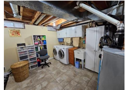
Pic. 27: Laundry / Utility room
