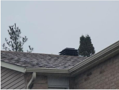
Pic. 4: Updated roof covering
