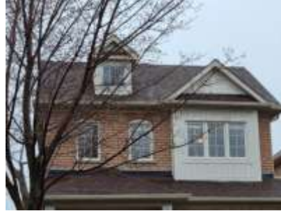
Pic. 2: Updated roof covering
