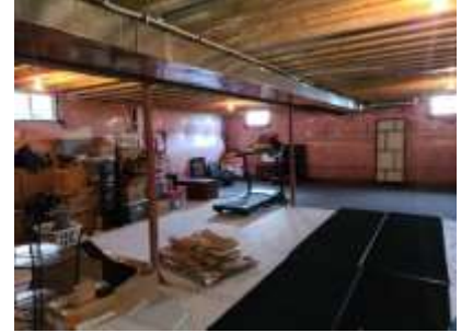
Pic. 30: Unfinished basement
