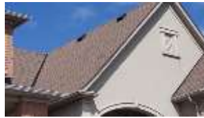
Pic. 2: Repaired roof covering
