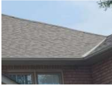
Pic. 2: Updated roof covering
