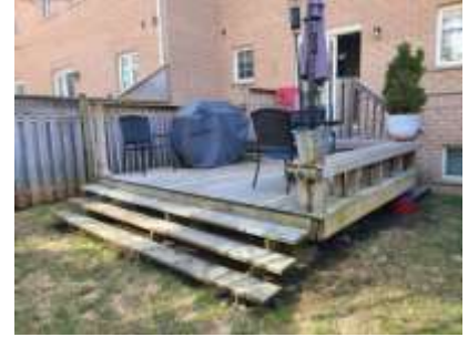
Pic. 6: Rear deck
