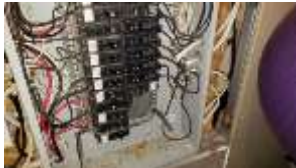
Pic. 41: 200 amp breaker panel
