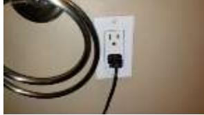
Pic. 38: Bathroom outlet should be GFCI protected
