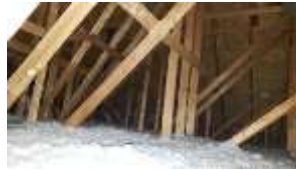
Pic. 11: Upgraded insulation level
