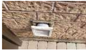
Pic. 3: Exhaust vent needs to be reset to the wall
