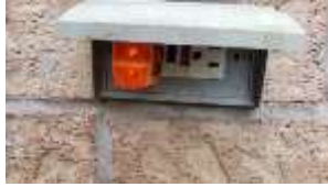
Pic. 6: Rear GFCI defective
