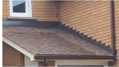
Pic. 2: Updated roof covering
