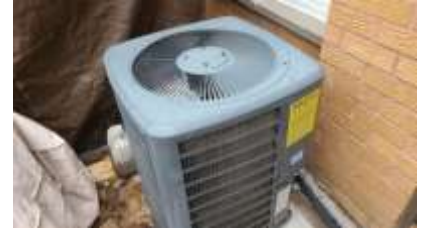
Pic. 6: Ac unit 2009A
