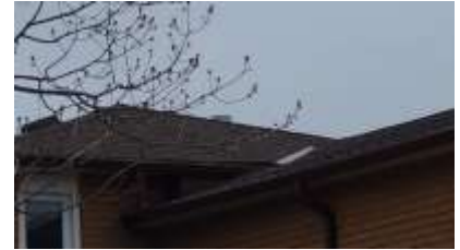
Pic. 3: Updated roof covering
