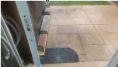
Pic. 22: Torn patio screen door
