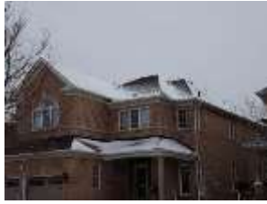
Pic. 2: Roof covering
