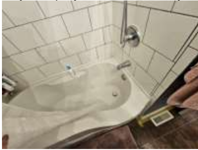
Pic. 16: 2 nd floor bathroom
