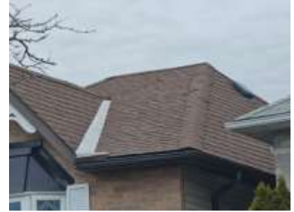
Pic. 3: Roof covering
