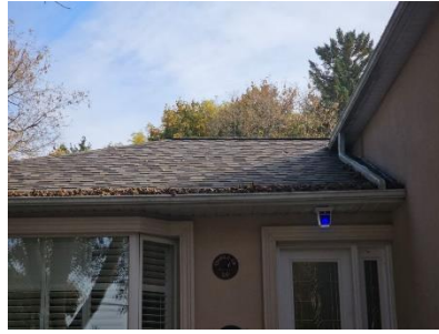
Pic. 2: Updated roof covering
