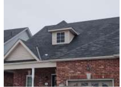
Pic. 3: Roof covering
