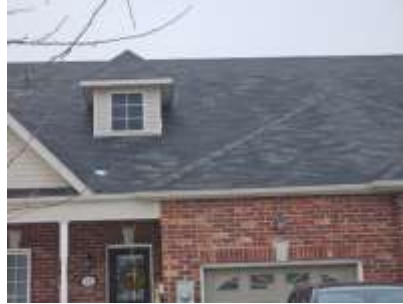
Pic. 2: Roof covering
