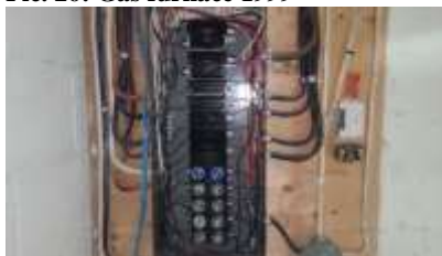
Pic. 29: 100 amp fuse panel with all copper wire
