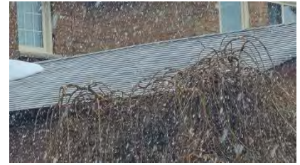
Pic. 3: Roof covering
