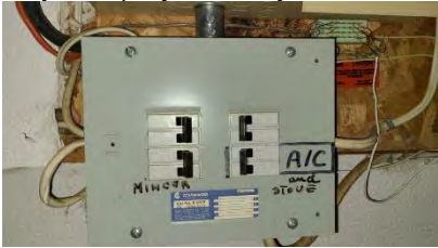
Pic. 37: Basement pony panel
