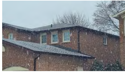
Pic. 2: Roof covering
