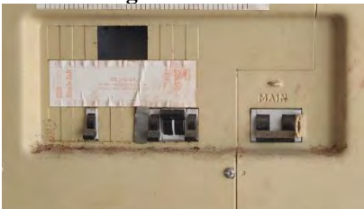
Pic. 10: Opening in the front of the panel needs to be sealed
