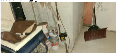
Pic. 43: Water main
