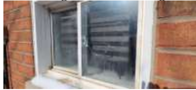
Pic. 5: Broken glass panel in basement Rec room
