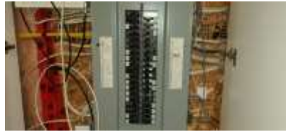
Pic. 35: 150 amp breaker panel
