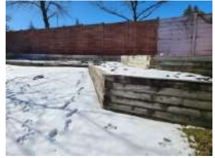
Pic. 3: Retaining wall
