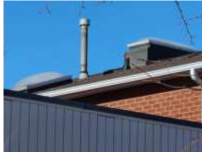
Pic. 2: Roof covering and skylights
