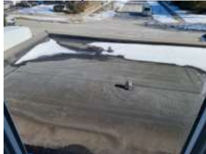
Pic. 8: Garage flat roof
