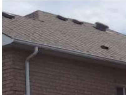
Pic. 2: Updated roof covering
