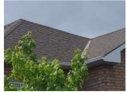
Pic. 3: Updated roof covering
