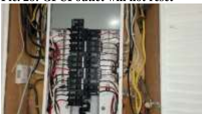
Pic. 31: 100 amp breaker panel with all copper wire
