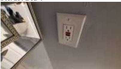
Pic. 28: GFCI outlet will not reset
