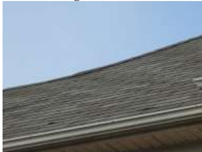
Pic. 8: Original roof covering
