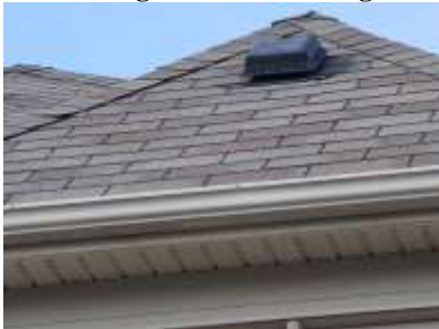
Pic. 7: Original roof covering
