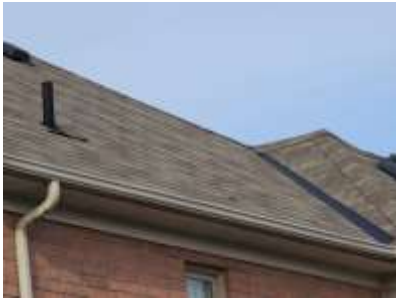
Pic. 4: Original roof covering
