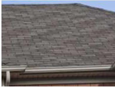
Pic. 2: Original roof covering
