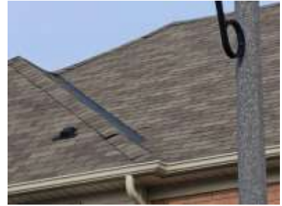
Pic. 3: Original roof covering
