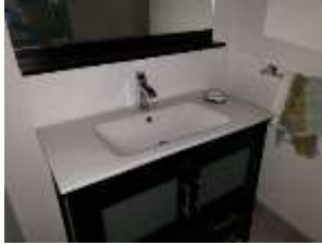
Pic. 29: Basement bath
