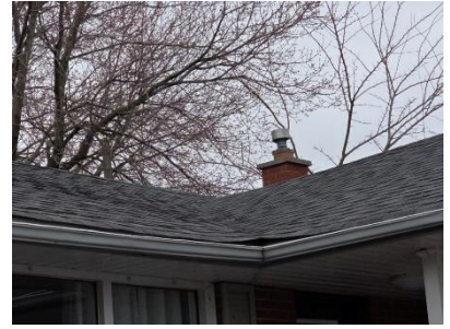
Pic. 3: Updated roof covering
