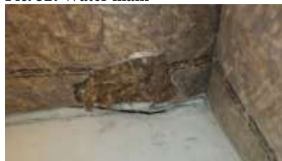
Pic. 35: Vapour barrier needs to be sealed
