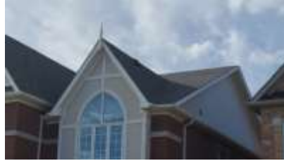
Pic. 2: Roof covering
