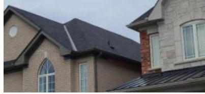
Pic. 2: Roof covering
