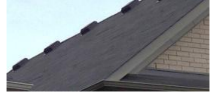
Pic. 3: Roof covering
