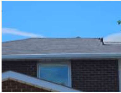
Pic. 2: Roof covering
