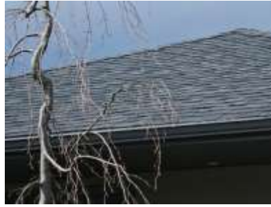
Pic. 2: Updated roof covering
