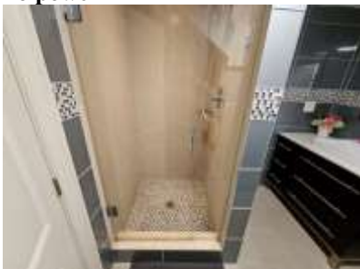
Pic. 28: Basement bathroom
