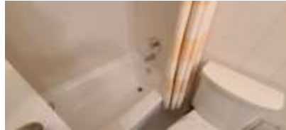
Pic. 11: 2nd floor bathroom
