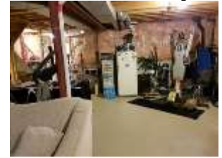
Pic. 24: Unfinished basement
