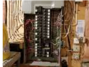
Pic. 27: 100 amp breaker panel with all copper wire
