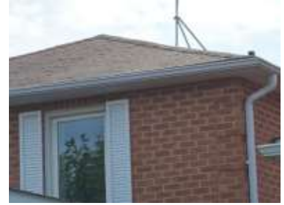
Pic. 3: Roof covering
