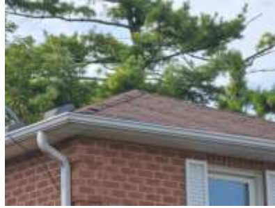
Pic. 2: Roof covering
