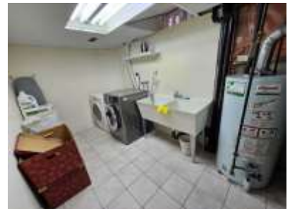
Pic. 27: Laundry room
