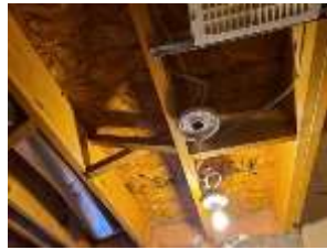
Pic. 27: Missing smoke detector in basement
