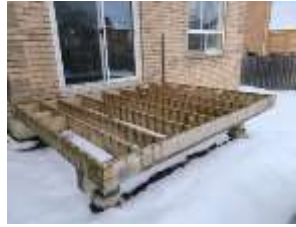
Pic. 3: Decking removed and needs to be replaced
