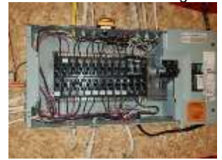
Pic. 28: 100 amp breaker panel with all copper wire
