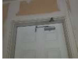
Pic. 7: Auto closer needs to be reconnected
