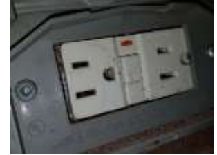
Pic. 8: Rear GFCIU outlet will not reset
