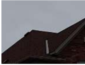
Pic. 2: Roof covering, one missing shingle tab at the top of the roof
