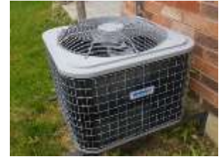
Pic. 4: AC unit
