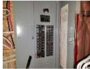
Pic. 31: 100 amp breaker panel with all copper wire
