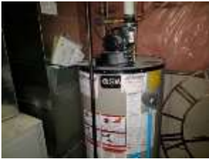
Pic. 29: Rental hot water tank
