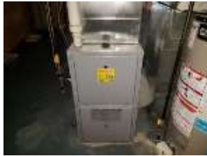
Pic. 30: High efficiency gas furnace
