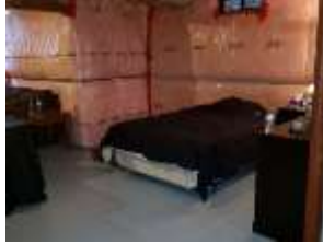
Pic. 26: Unfinished basement
