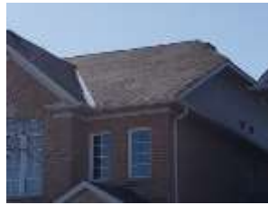
Pic. 2: Original roof covering
