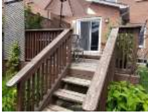
Pic. 5: Rear deck
