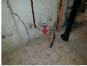
Pic. 30: Water main
