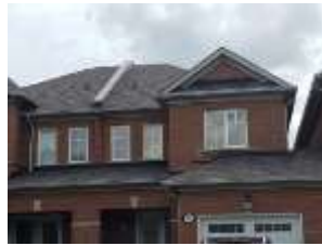
Pic. 2: Updated roof covering
