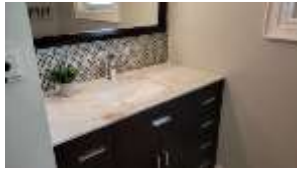
Pic. 26: 2 nd floor bath
