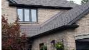
Pic. 2: Updated roof covering
