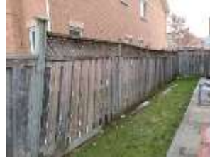
Pic. 7: Fence needs repairs
