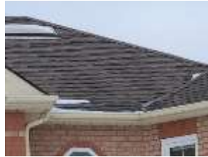
Pic. 2: Roof covering
