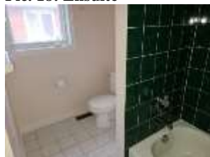
Pic. 22: 2 nd floor bath
