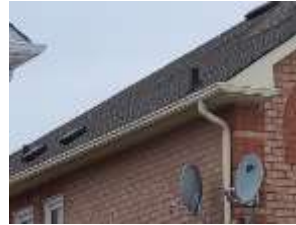
Pic. 3: Roof covering
