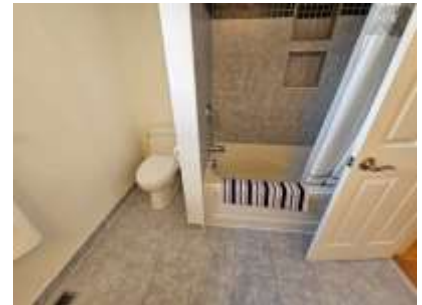
Pic. 21: 2 nd floor bath
