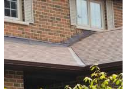
Pic. 3: Roof covering
