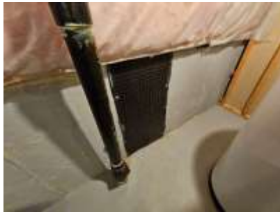
Pic. 35: Foundation repair
