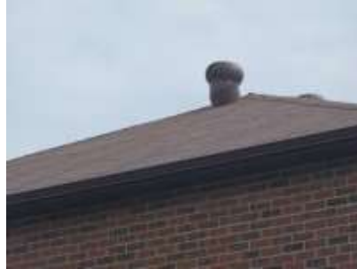
Pic. 5: Roof covering
