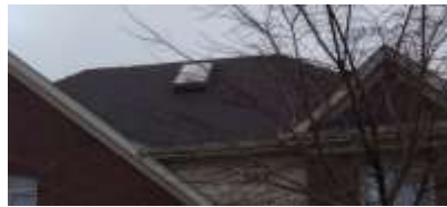
Pic. 2: Original roof covering
