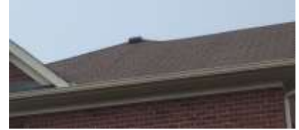
Pic. 6: Original roof covering
