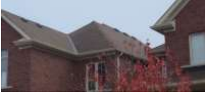
Pic. 4: Original roof covering
