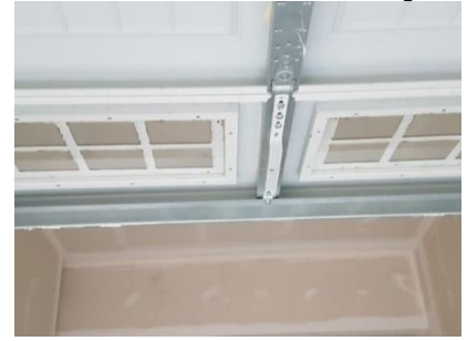
Pic. 15: Garage door, no opener
