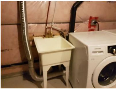
Pic. 52: Laundry area
