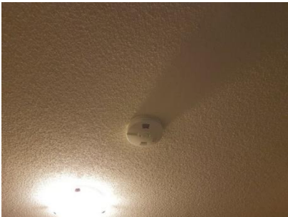
Pic. 31: 2 nd floor smoke / co detector
