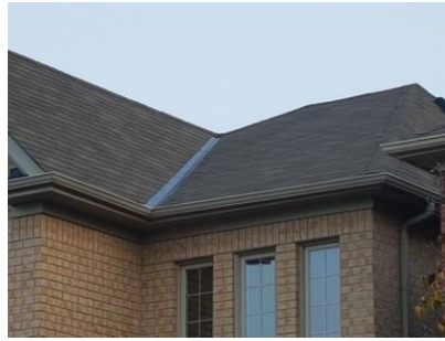
Pic. 2: Front roof covering
