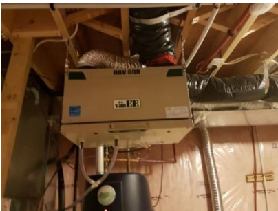
Pic. 58: Furnace HRV unit
