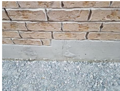
Pic. 5: Typical foundation crack
