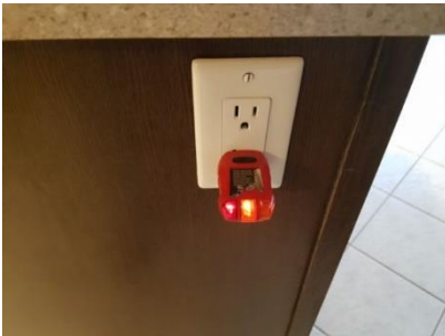
Pic. 43: Kitchen outlet end of island wired incorrectly and needs repair
