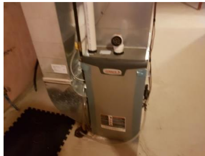
Pic. 59: High efficiency gas furnace
