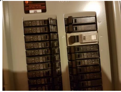
Pic. 62: Proper ARFC breaker for bedroom outlets
