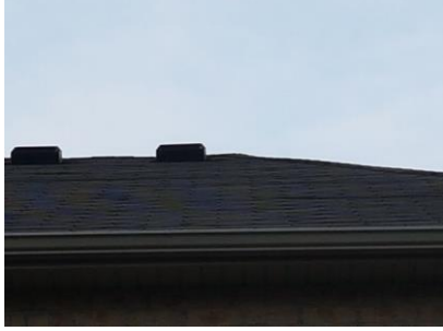
Pic. 13: Rear roof covering
