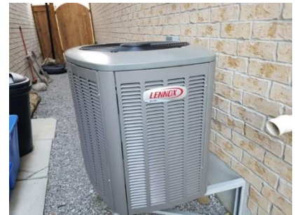
Pic. 9: AC unit
