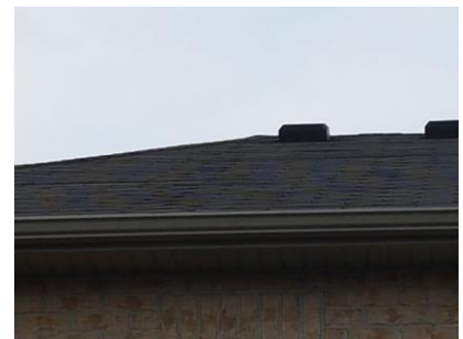
Pic. 12: Rear roof covering , one missing shingle tab, repair /replace accordingly
