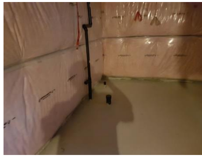
Pic. 53: Basement: rough in bathroom
