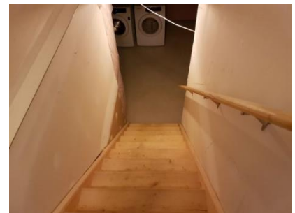
Pic. 48: Basement stairwell
