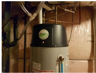
Pic. 56: Hot water tank
