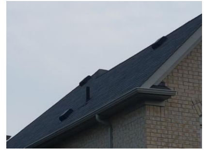
Pic. 3: Side roof covering
