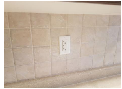
Pic. 42: Kitchen GFCI outlet
