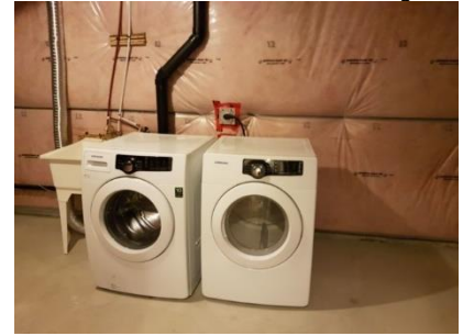
Pic. 51: Laundry area
