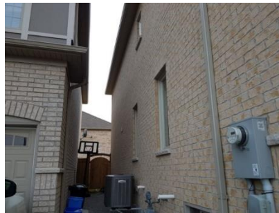
Pic. 8: Side view
