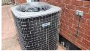
Pic. 6: AC unit 2006
