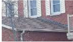
Pic. 3: Updated roof covering
