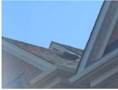
Pic. 2: Updated roof covering
