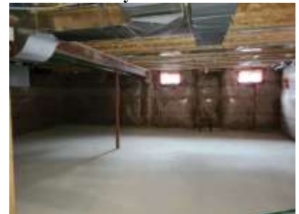
Pic. 27: Unfinished basement
