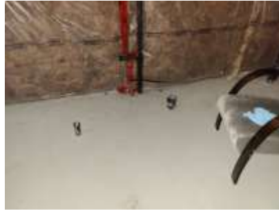
Pic. 32: Bathroom rough in
