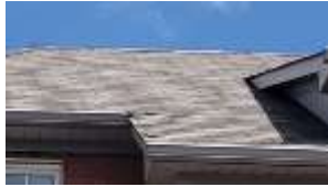
Pic. 2: Original roof covering
