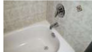
Pic. 15: 2 nd floor bath
