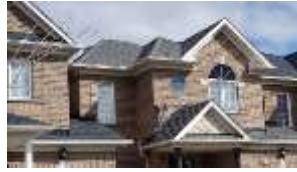
Pic. 2: Updated roof covering
