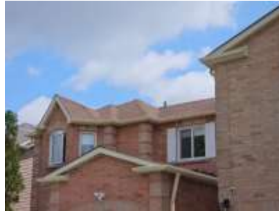
Pic. 2: Roof covering
