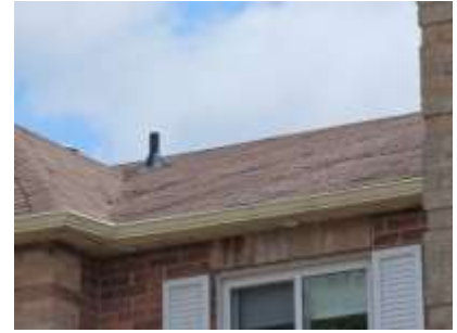
Pic. 3: Roof covering
