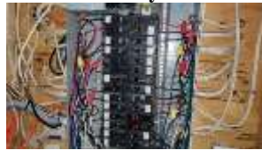
Pic. 31: 100 amp breaker panel
