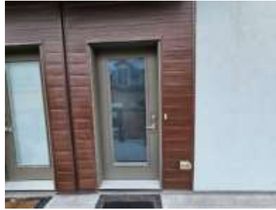
Pic. 2: Front door on second level
