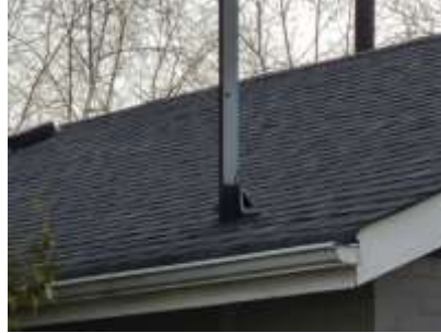
Pic. 2: Updated roof covering
