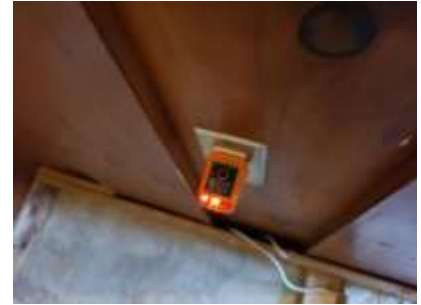
Pic. 21: Reverse polarity outlets in Rec room
